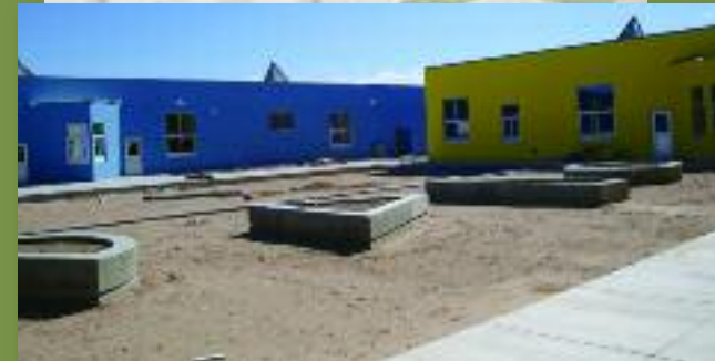
Helen Cordero Primary School will be LEED Silver certified and will include Ground Source Heat Pumps HVAC system.
